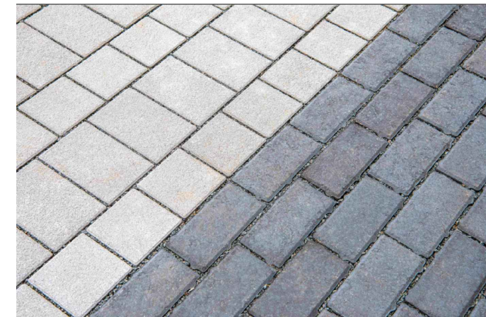
EXAMPLE PERMEABLE PAVING
