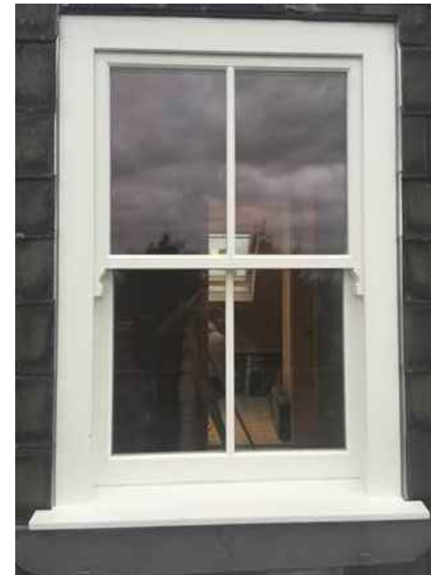
EXAMPLE WHITE TIMBER SASH WINDOWS FRONT ELEVATION
